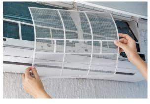
Fig. 5.5.3: Taking the filter out
