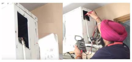
Fig. 5.5.11: Measuring voltage and current
