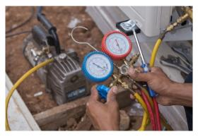
Fig. 5.5.12: Measuring pressure using manifold gate
