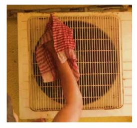
Fig. 5.5.6: Cleaning of outdoor unit
