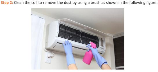
Fig. 5.5.4: Cleaning the dust
