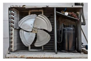
*Fig. 5.5.13: Parts of outside unit* **Step 5:** Remove fan motor and cover the outdoor connection box.
