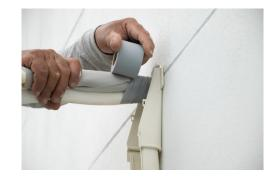
Fig. 5.4.23: Wrap piping joints with insulating tape
