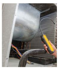
Fig 4.10.17: Leak detection using electronic refrigerant detector
