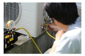
Fig. 5.4.22: Remove air and humidity
