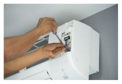
Fig. 5.5.7: Remove the front cabinet
